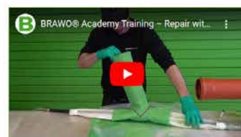
BRAWO® Academy Training – Repair with BRAWO® connection collars
